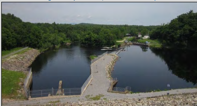
Figure 7.4 Hopkinton Dam, Contoocook
