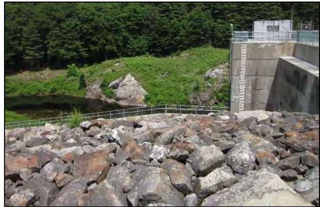
Figure 7.9: Rocks Used for Erosion Control Blackwater Dam, Webster
