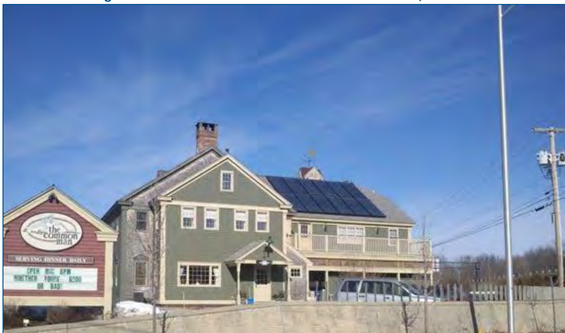
Figure 9.7: Common Man Hot Water Solar Installation, Concord
