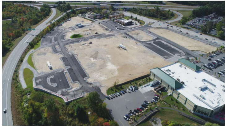
Market on Main Construction, 2017. Photo: Derek Shooster
